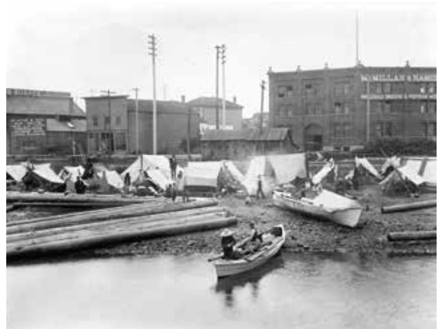
First Nations people camped on Alexander Street beach at the foot of Columbia Street, circa 1898
